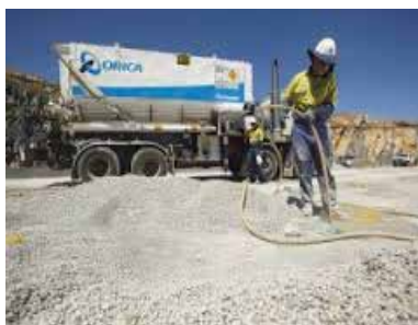
Figure 48: Bulk loading of ANFO
