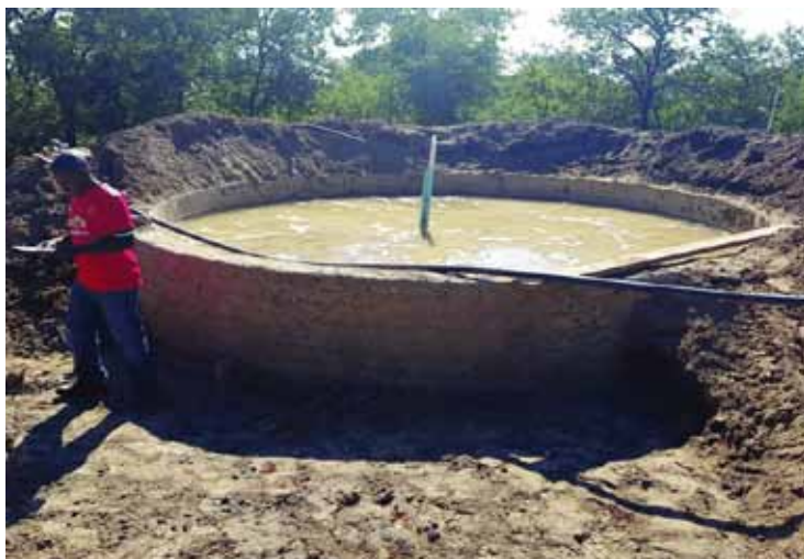
Figure 105: Typical leach tanks used in ASM
