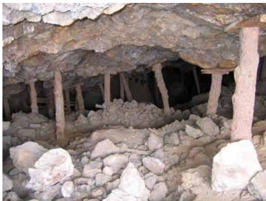
Figure 68: Timber props in a stope (source: www.mcrocks.com )
