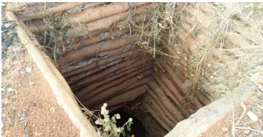
Figure 62: Timbered shaft
