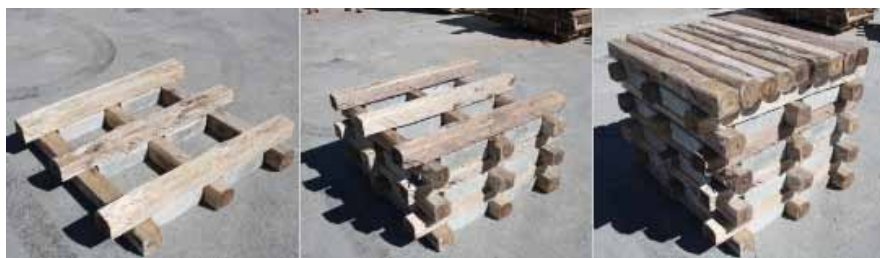
Figure 69: Construction of mat packs
