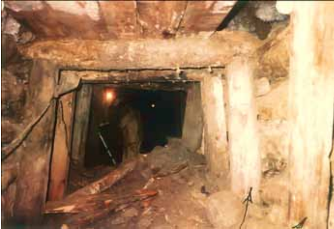
Figure 70: Timber sets in a drift (Source: www.goldrushexpeditions.com )
